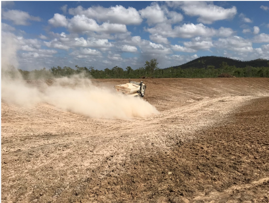
Plate 3 Direct application of gypsum on this site at a rate of 18t/ha was sufficient to bring soil sodicity down to approximately 6% ESP (Source: Damon Telfer, Fruition Environmental)
