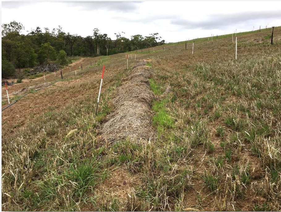
Plate 2 The use of hay mulching on mid-batter faces may have value as a temporary flow retardant where batter lengths result in significant catchment areas (Source: Glenn Dale, Verterra)
