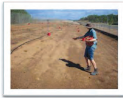
Photo 7. Direct seeding native grasses by hand can help stabilise a modified bank. Hand sowing is only practical for small sites such as this one.
