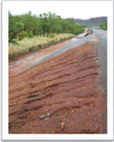
Photo 3. Reducing the risk of soil erosion is a major challenge due to intense rain storms that occur during the wet season. Rills have already formed on this steep bank.
