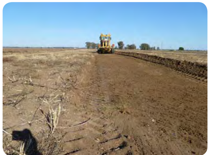
Our year one Plains savannah restoration has been scalped to a depth of 200mm.
