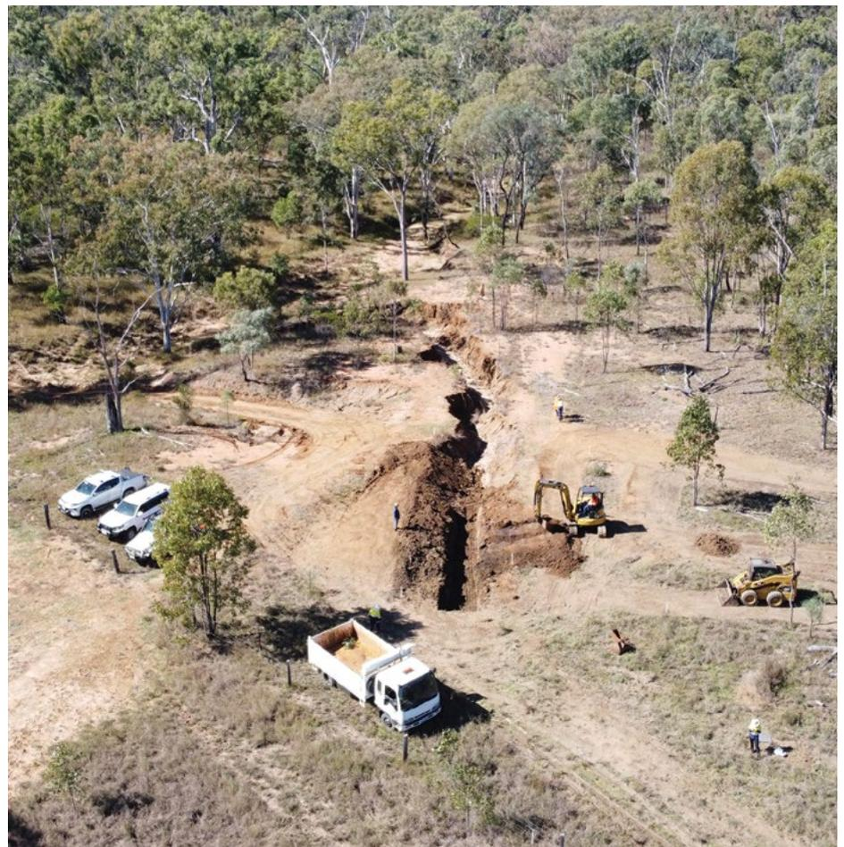
Earthworks under way to remediate gully erosion at Lily Creek in Central Queensland.
