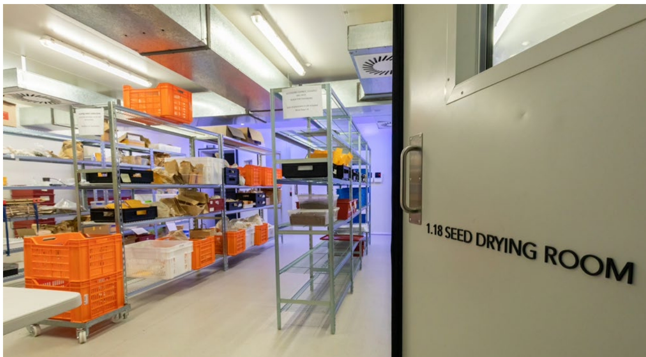
Figure 17. A purpose-built seed drying room, with controlled temperature and relative humidity. (Photo: N. Emery)
