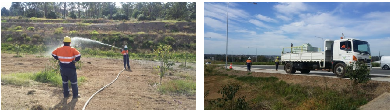
Figure 11. Hydroseeding of road batters. (Photos: P. Gibson-Roy)
