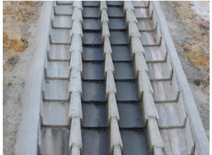
**Stabilised drain outlets** reduce the force of the water coming out of the drain to minimise erosion.
